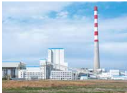
Plant with air-cooled condensers at Keyouzhong thermal power plant (2 x 300 MW), China
