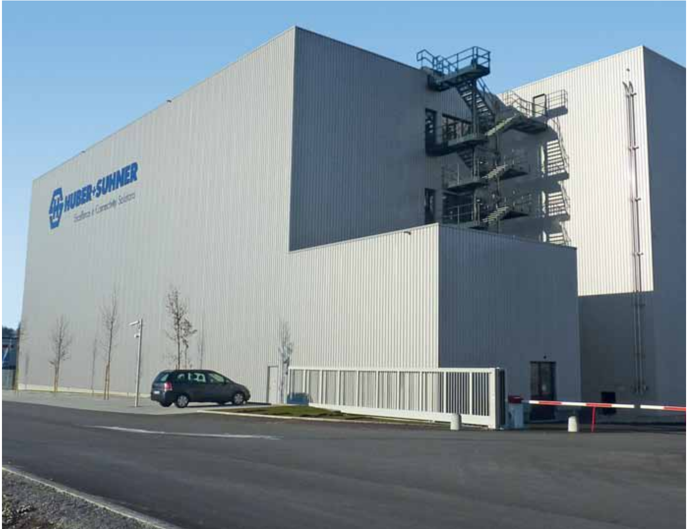
New construction of a mixing facility for Huber+Suhner in Pfäffikon near Zurich
